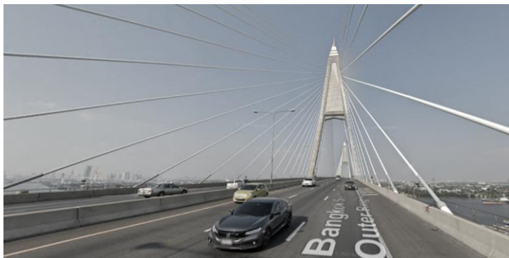
堪恰納披色大橋 - 斜拉橋 Kanchanaphisek Bridge
